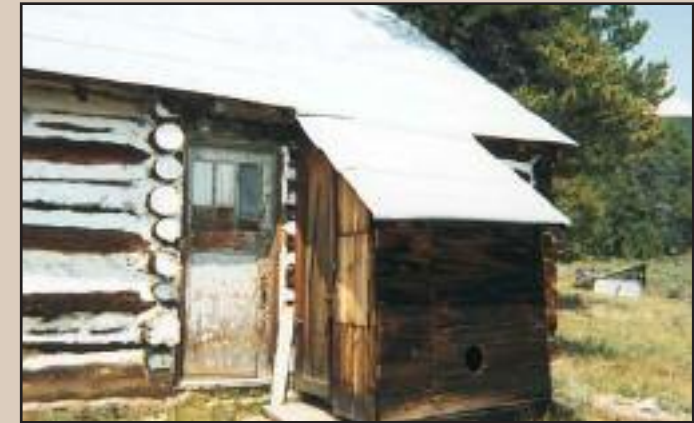
Attached Union Park facility shows port for waste removal.
